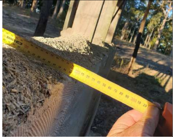
Photo 2: wall 200mm thick
