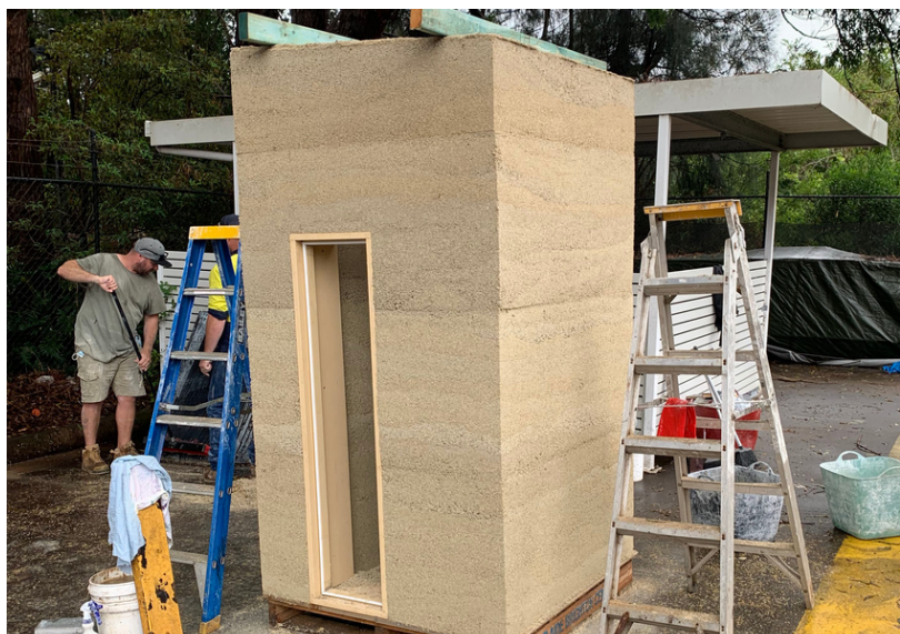
Getting ready for the roof to be put onto the first of the 4 builds happening at UTS, the Hemp build using cast-in-place or in situ construction.
