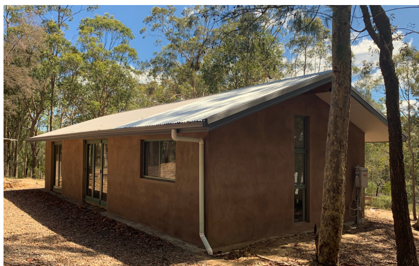
Hemp retrofit, NSW Central Coast. Situated on a BAL 29 bush block on the Central Coast hinterland, what was originally a timber framed, fibre cement clad build with gyprock interior walls was retrofitted with hemp to improve thermal performance and fire safety.
